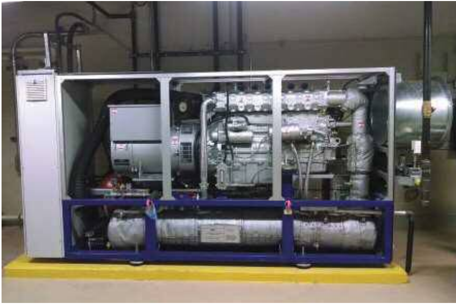
A combined heat and power (CHP) system supplied by MTU Onsite Energy and installed by distributor W.W. Williams yielded significant savings in its first year of operation at an Ohio high school and recreation center.
