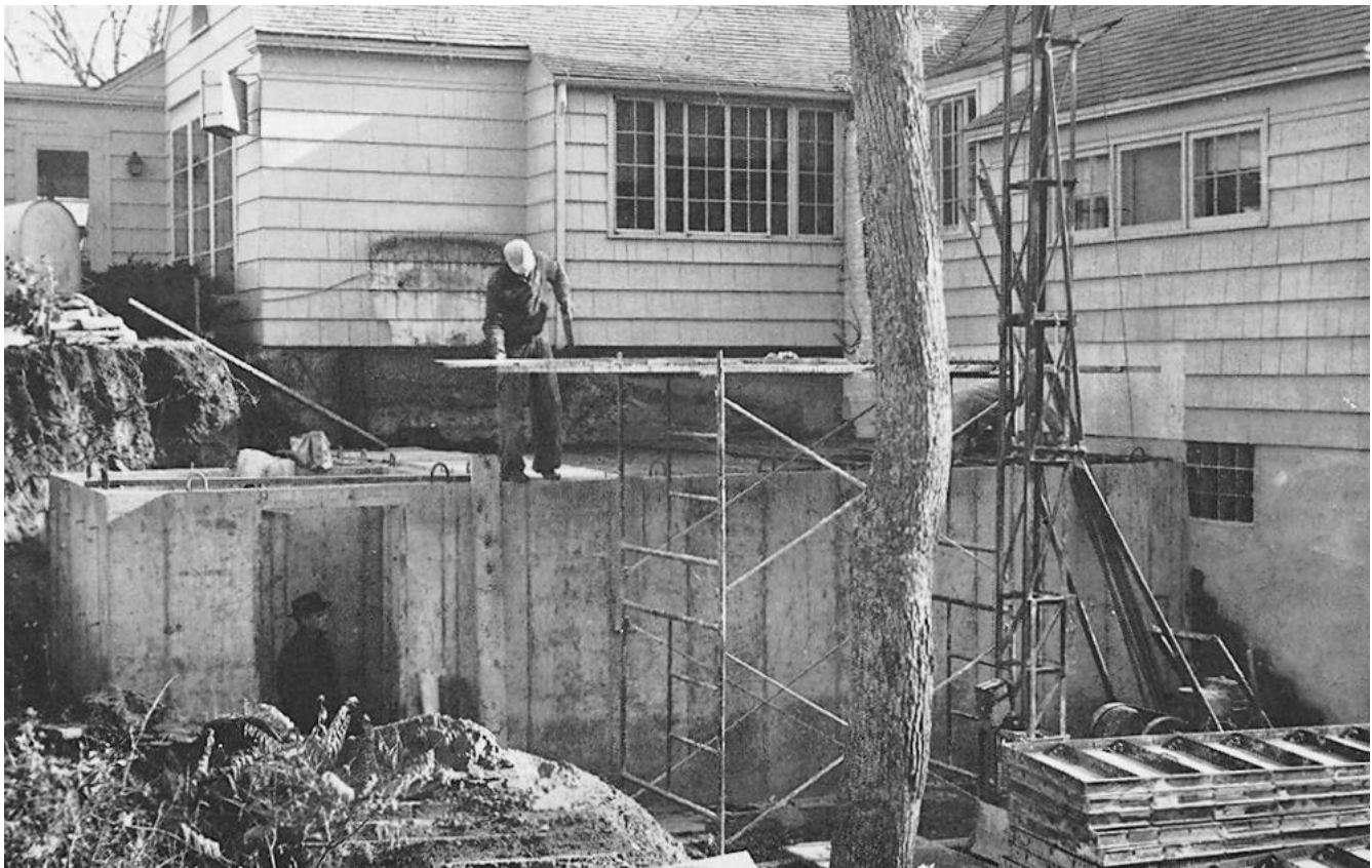
Shown here is a fairly monolithic underground survival shelter being constructed in Excelsior, Minnesota.
