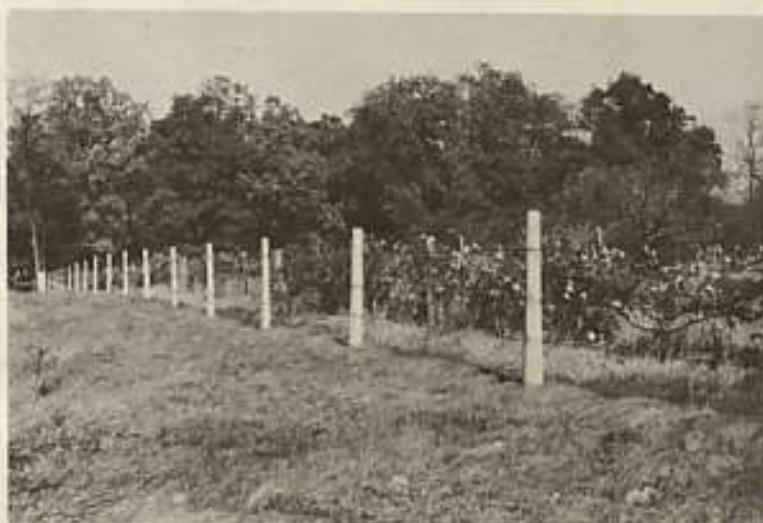
These concrete posts erected in 1914 on the Iowa Experiment Station farm at Ames, Iowa, were 25 years old when this photograph was taken. They will continue to give trouble-free service for many years.
