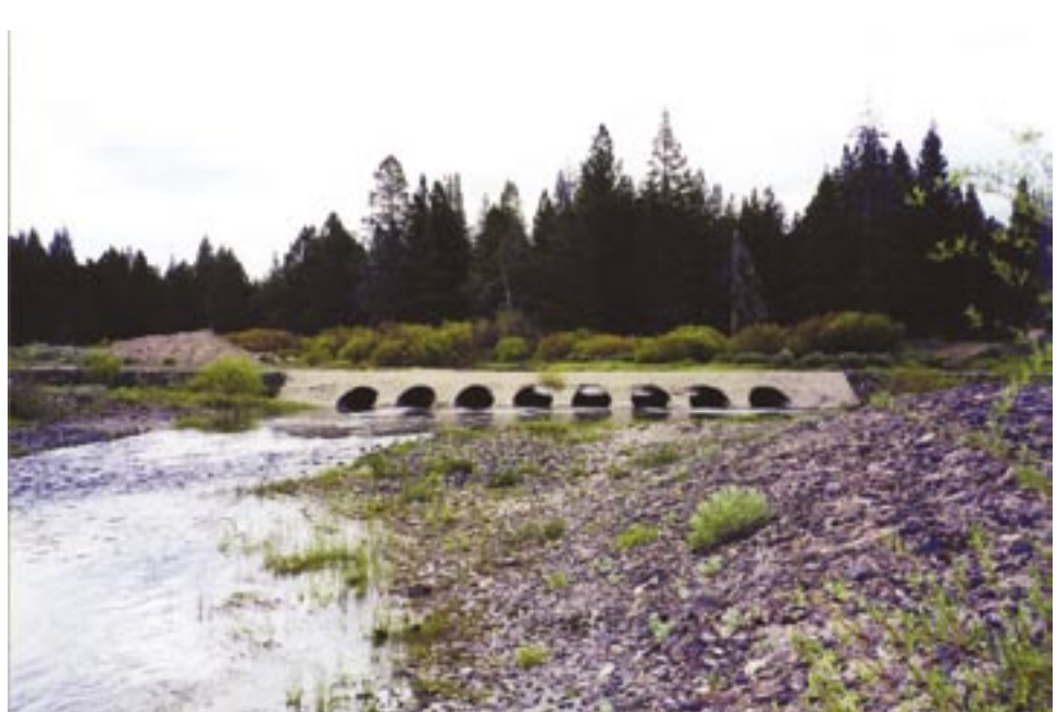
Figure 5.13a—Murdock vented ford, Plumas National Forest, California looking upstream (note excavated sediment upstream of ford).
